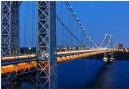
George Washington Bridge
